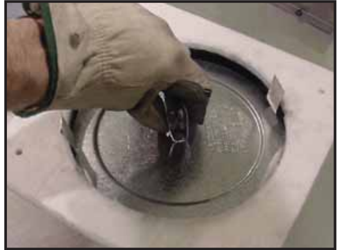
Figure 7.4 Fold the center parts of the retaining band up and use to remove the vent cap.
